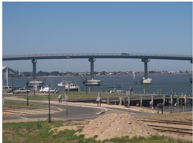
Hindmarsh Island Bridge | Construction was completed in 2001
